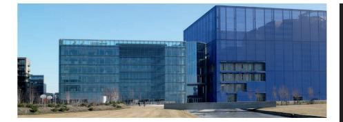
facing the outer facades while others face the inner courtyards. Together, the flexible arrangement encourages creativity and interdisciplinary cooperation. The outer skin is a beautiful but simple transparent envelope consisting of tilted glass louvres. Partly open courtyards within are an integral part of the building's naturally ventilated climate and environmental strategy and add a distinctly green character.
