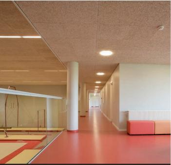
BBP Arkitekter A/S appreciates that they have been able to provide a smooth ceiling surface with integrated lighting from Troldtekt. The gym itself has been fitted with transversal armatures while the round ones are perfect for
